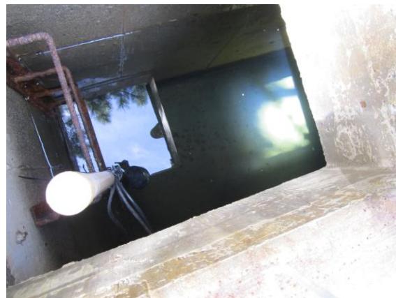
Upper reservoir interior
