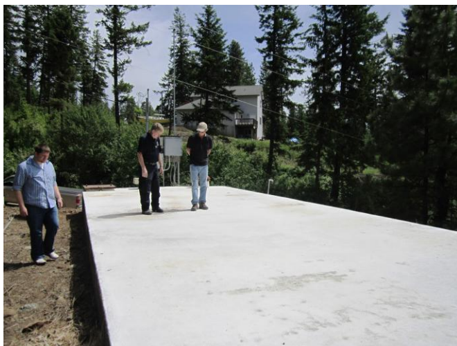
30,000 gallon Midway reservoir
