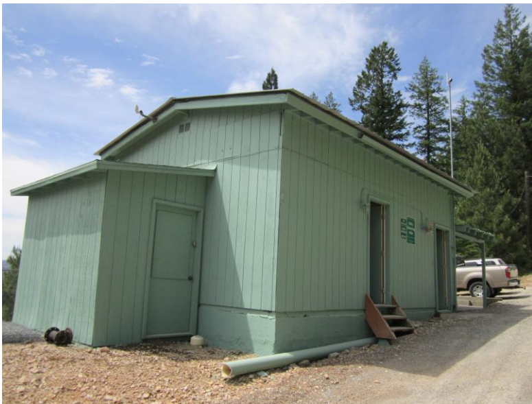
Filtration treatment building (contact chamber below)
